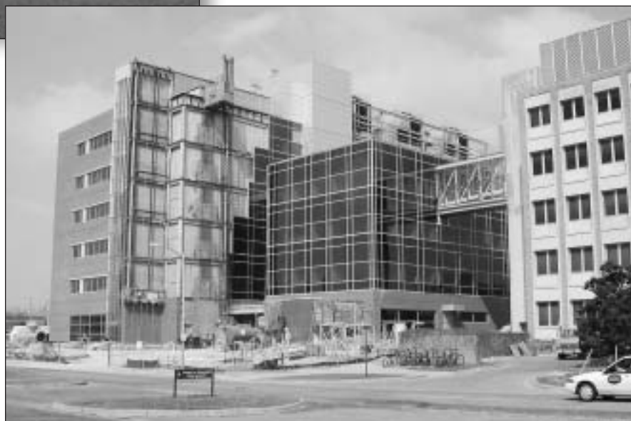
Status in March, 2001.
