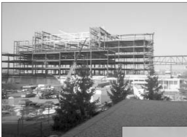
Status in March, 2000.
